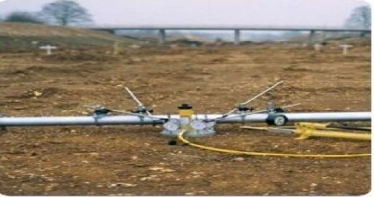
Plate Bearing Test
